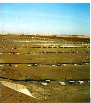
FlexAir™ high capacity tube and disc diffusers – well suited for the most rigorous coarse bubble applications requiring the utmost in system reliability.
