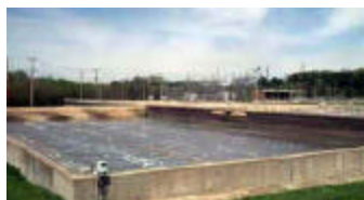
2.5 million gallon in-line equalization basin
