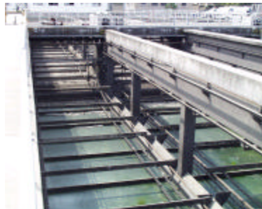
Empty Primary Settling Basins
