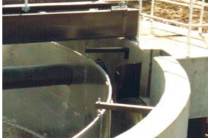
The Spiraflo's influent and effluent pipes are installed above the tank floor reducing the depth of excavation.
