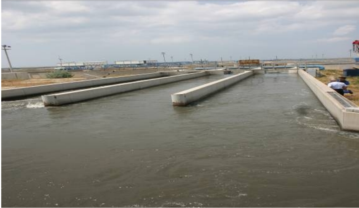
Activated sludge basins
