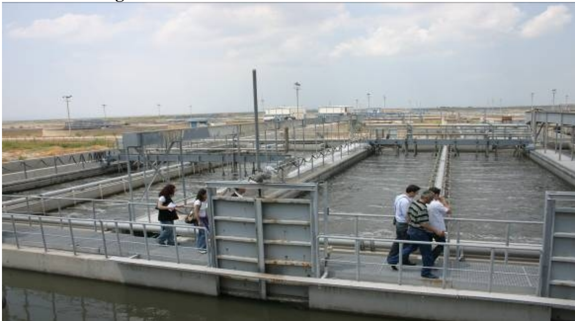
Activated sludge basins
